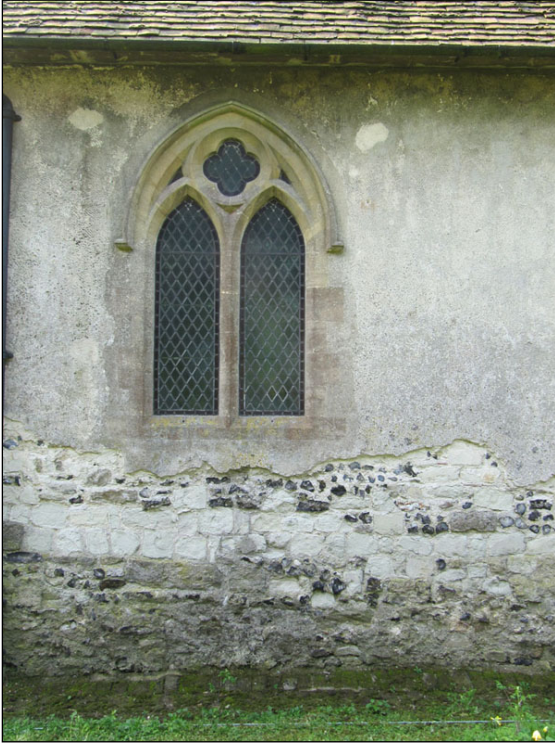
Fig 3: The north wall with infill of the gap created by the tower collapse. The window is modern (note the falling away of the render).
