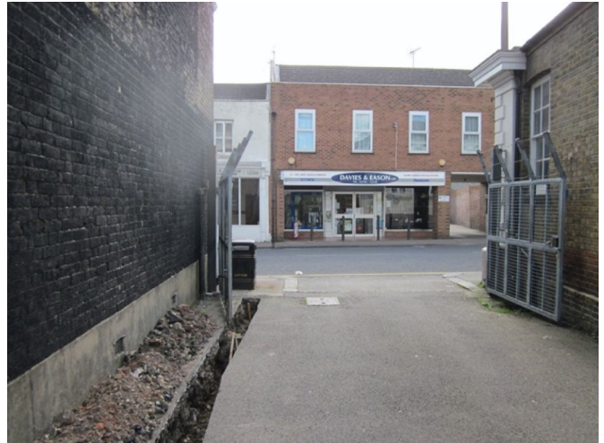
View of the trench towards Preston Street.
