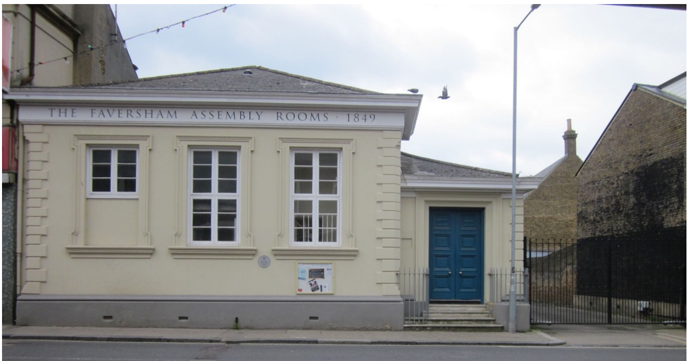
The newly renovated Faversham Assembly Rooms
