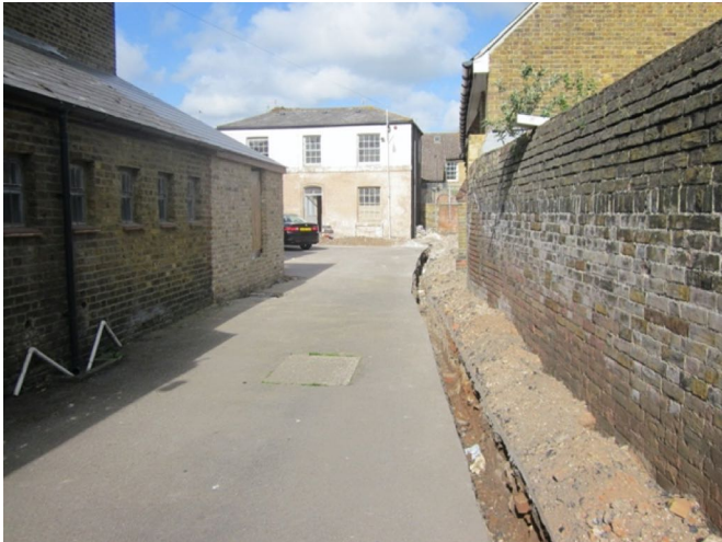
View of the services trench towards the Drill Hall Cottage.
